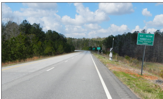
Section N11 at the NCAT Pavement Test Track, shown above, is a warm-mix asphalt section made with 50 percent reclaimed asphalt pavement.
