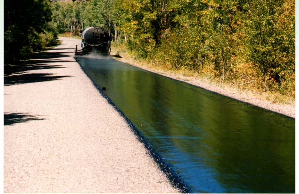
Distributor outrunning the chip spreader
