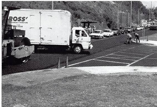
ABOVE: FRESHLY LAID SUPERPAVE WITHSTANDS TRUCK CROSSING
