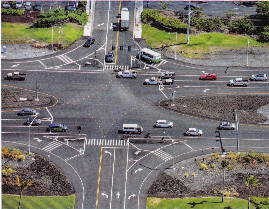
Completed improvements for the Hulikoa Drive intersection provided access to the Kohanaiki Resort and Kohanaiki Industrial areas.
