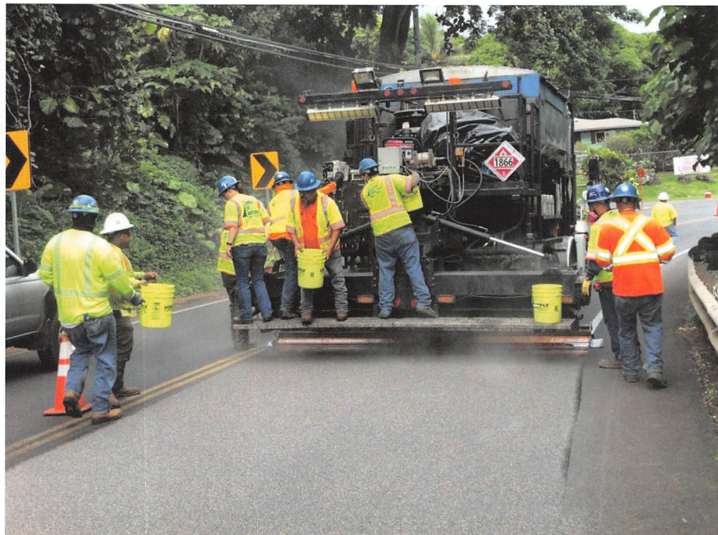
HFST application on Kamehameha Highway in Waiahole PHOTO COURTESY HDOT
