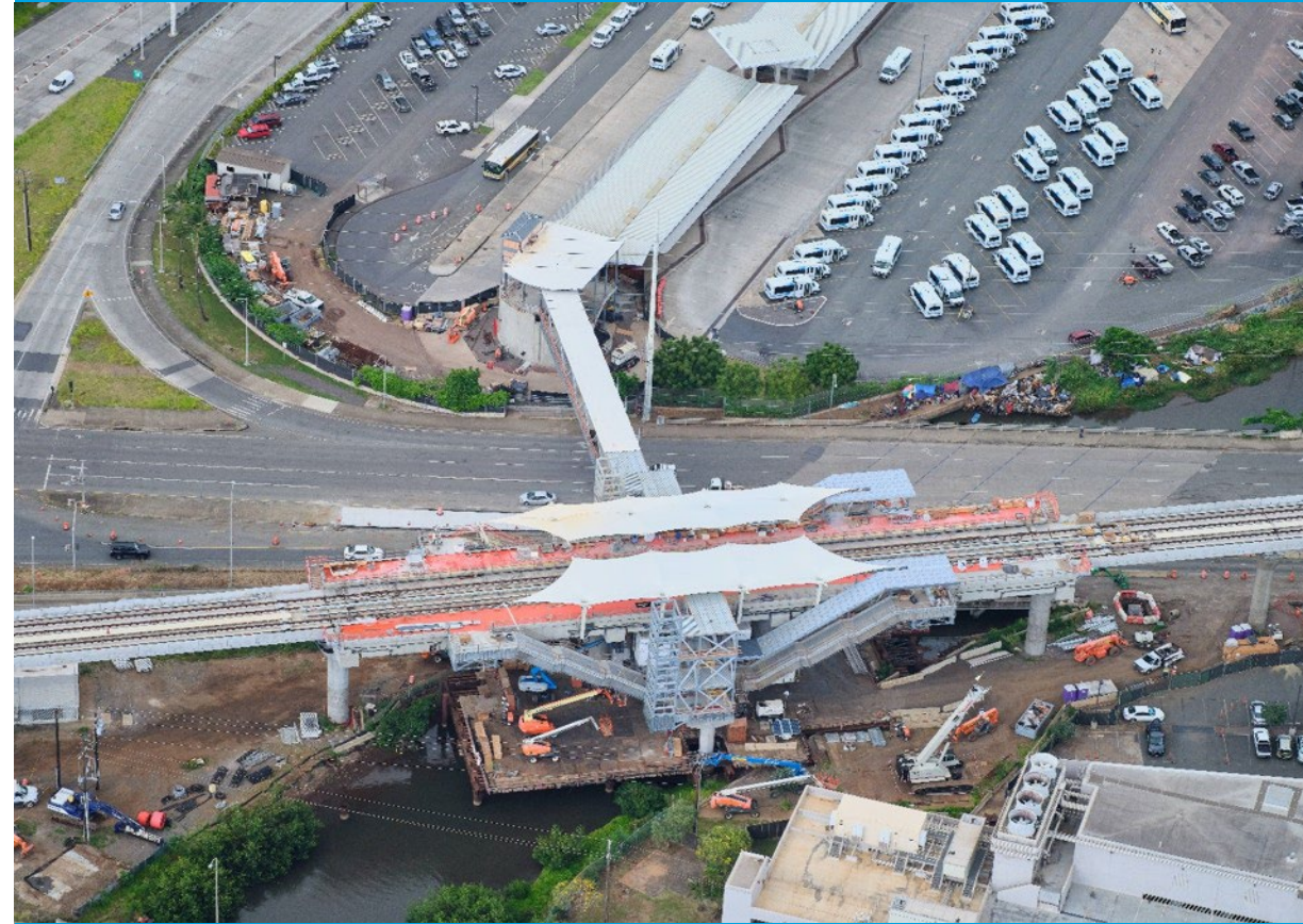
Pedestrian bridge over Kamehameha Highway
