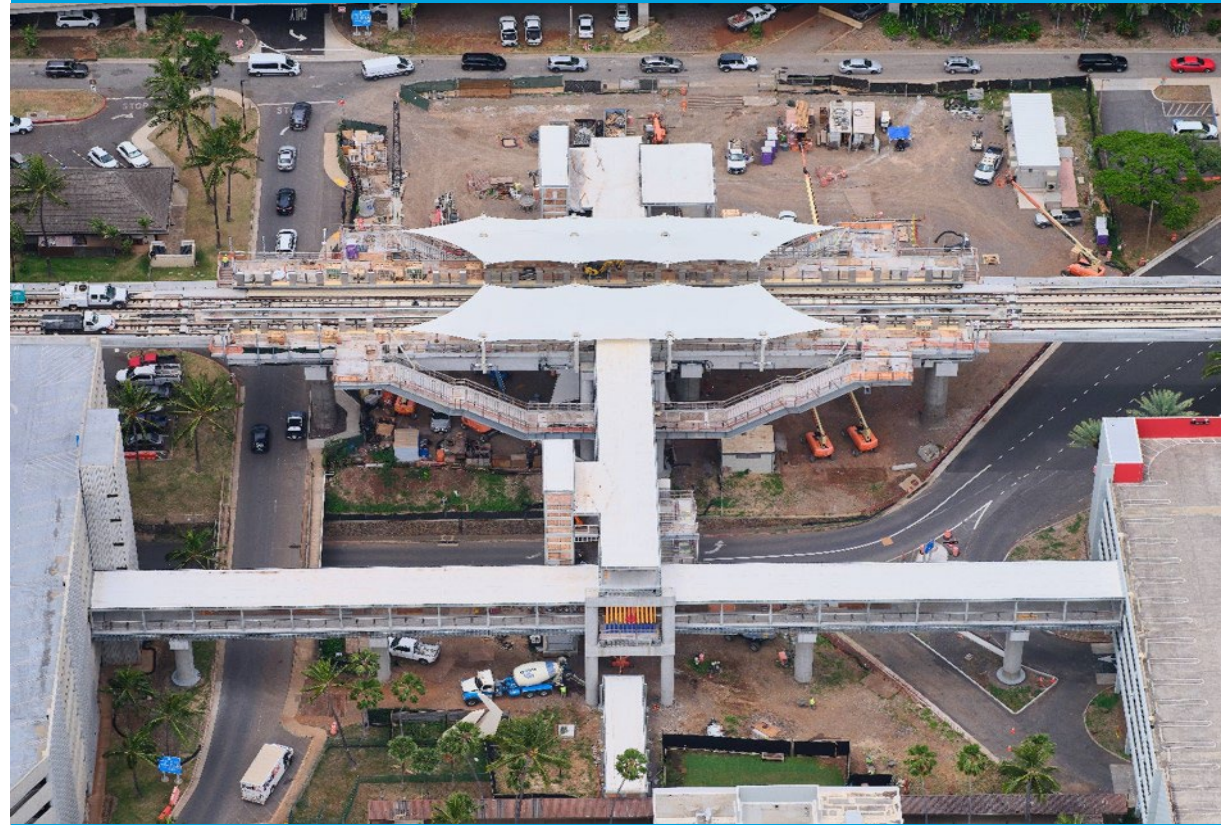
Stairway and platform level work is ongoing
