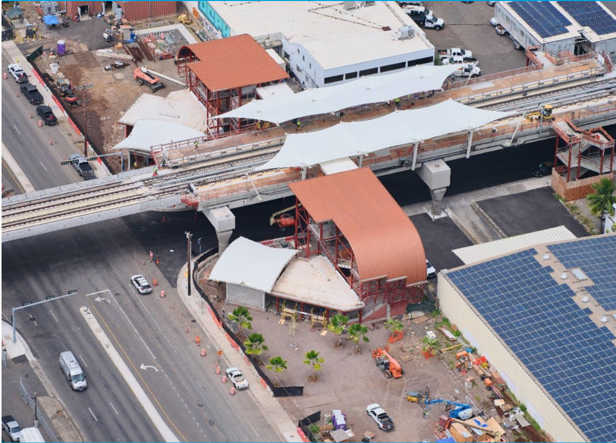
Paving activities underway restoring roadways and driveways
