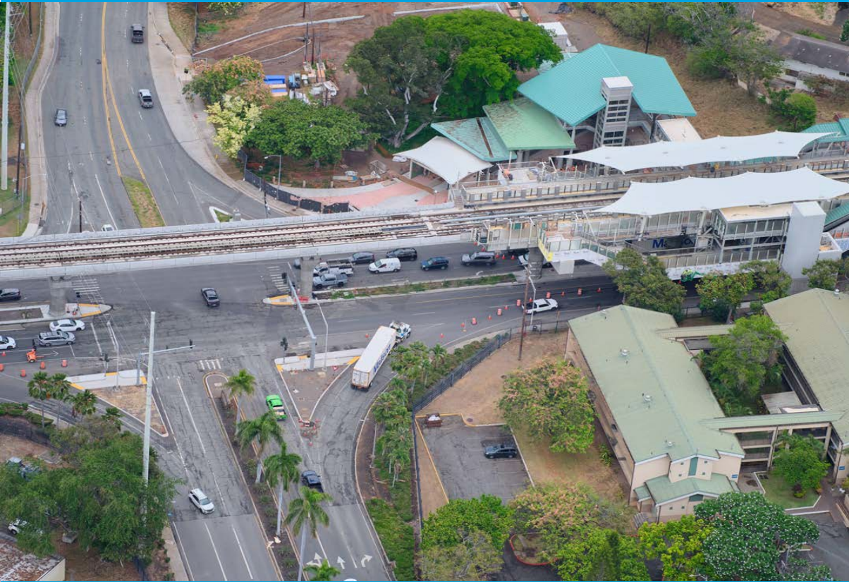
Road work working with traffic underway
