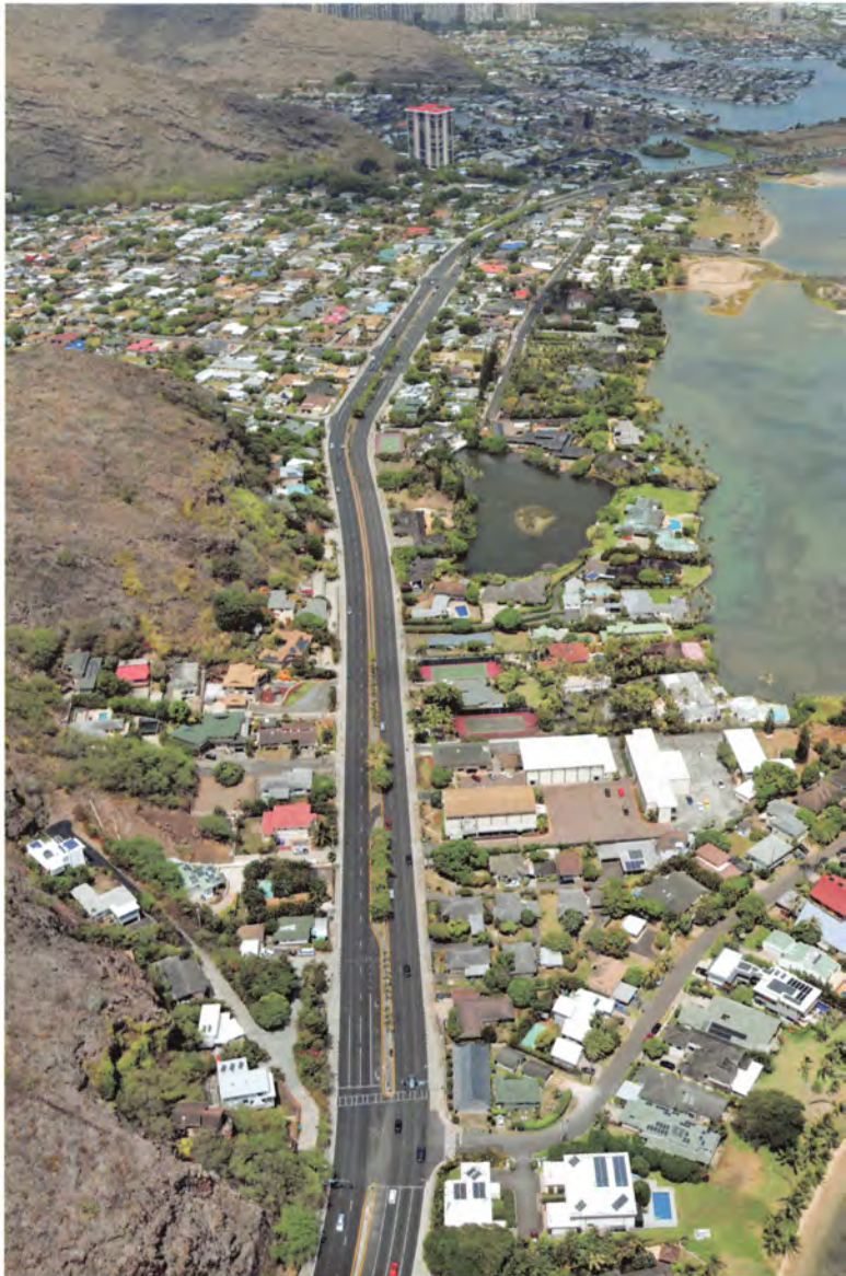
Grace Pacific is resurfacing Kalaniana'ole Highway.
