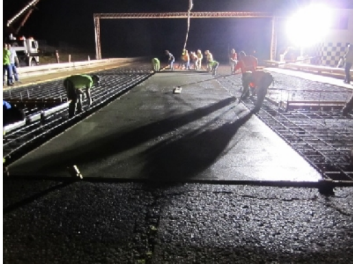
Figure 3 – Pouring of concrete launch Pad
