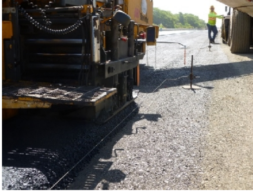
Figure 5 – Pavement installed using the tried and true “String Line” method
