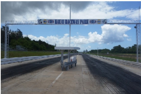
Figure 9 – Completed Track Improvements (Concrete Launch Pad)
