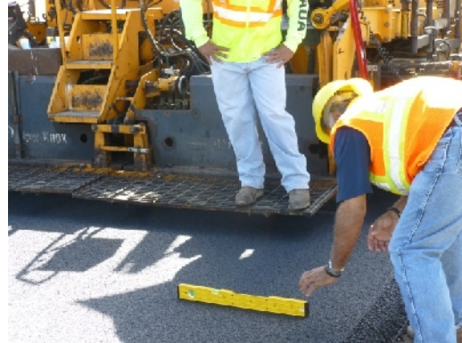
Figure 4 – Checking loose AC with 3-foot digital level prior to rolling.
