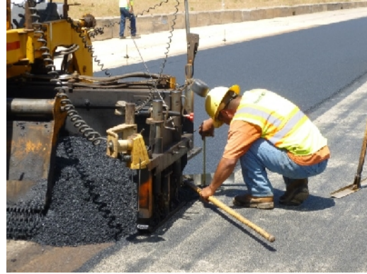
Figure 6 – Verifying pavement thickness prior to rolling.
